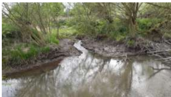
Reduced river levels on the Rhee in April 2019, showing Hoffers Brook entering the Rhee after completion of the removal of the weir at Harston Mill in March 2019 © Rob Mungovan.
