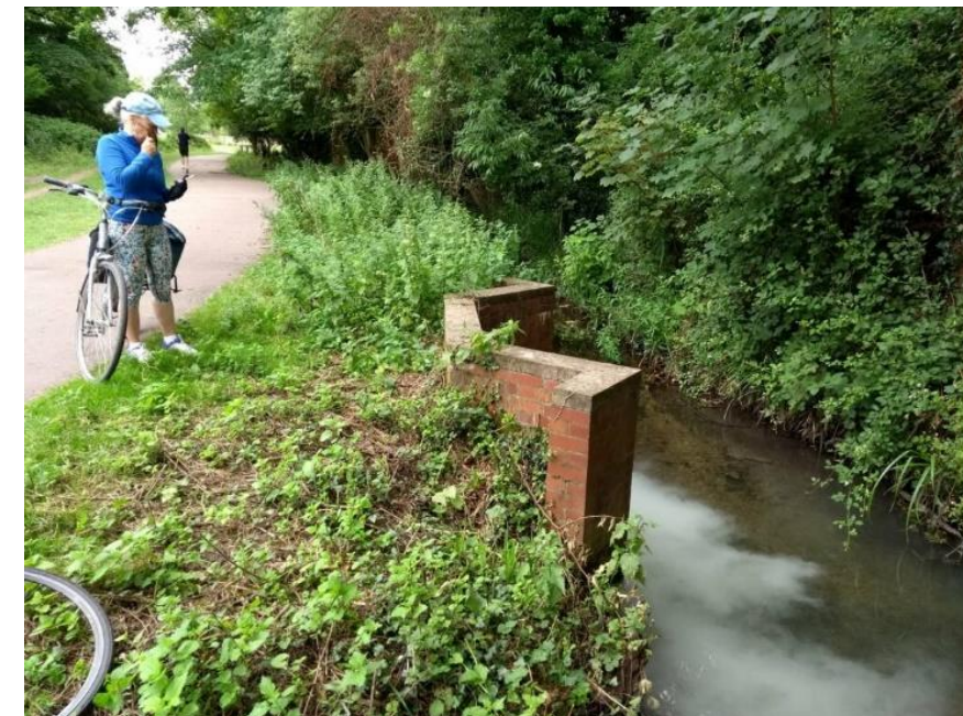
An outfall on Vicars Brook
