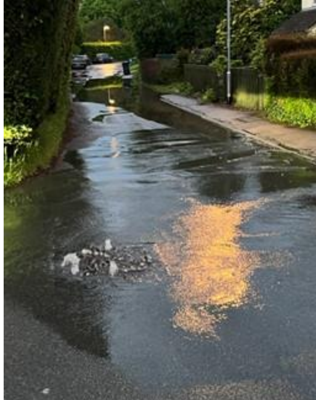
A “spill” at Harston pumping station releasing diluted sewage into the street at Button End
