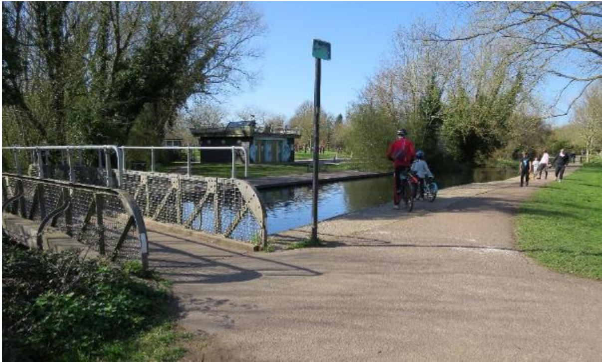
40. The 50m length of Snobs' Stream downstream of the footbridge has a concrete base at a depth of about 900mm and was where youngsters were taught to swim before the Learner Pool was built in the 1970s. The Learner Pool struggles with the number of children wanting to use it during peak times. Might this section of Snobs' Stream again be that step between the paddling pool and the river for young families gaining confidence in swimming? The public toilets are visible between the bridge and the signpost and the paddling pool is beyond.
