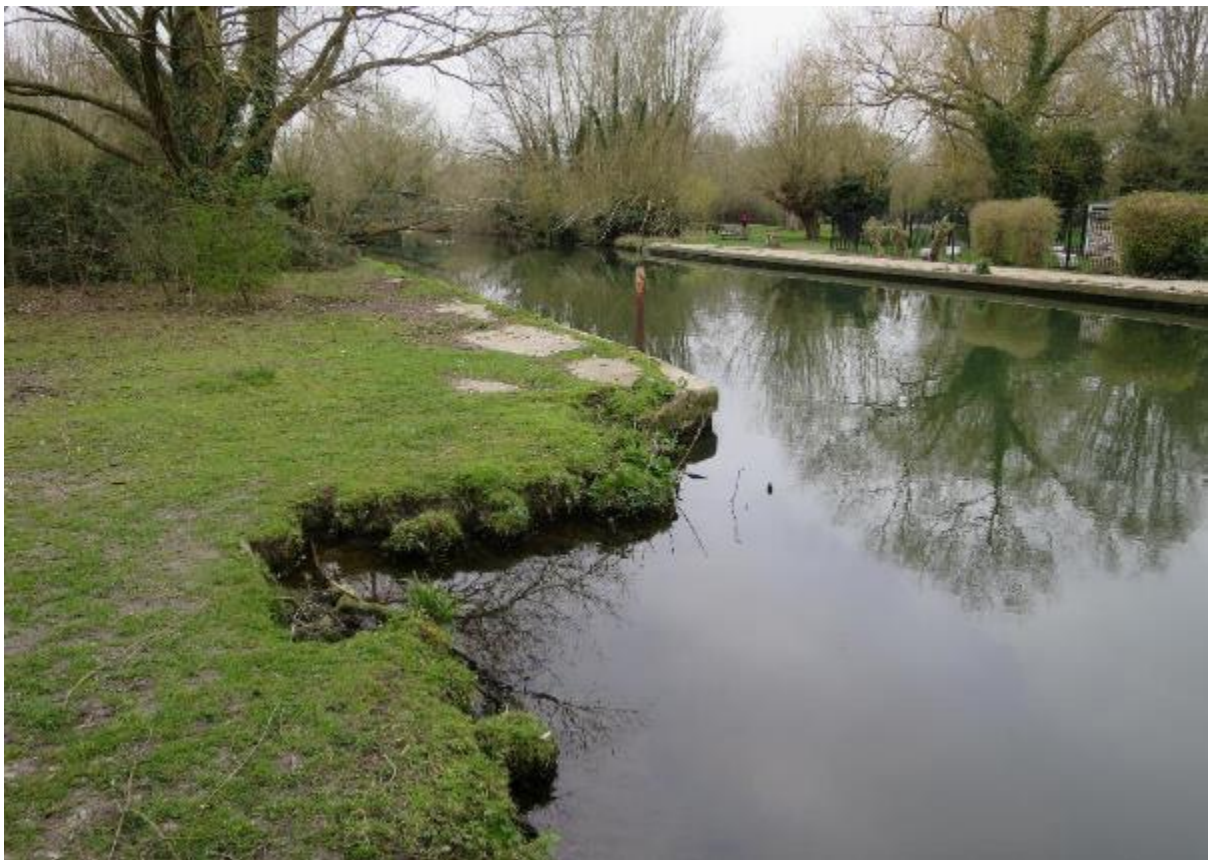
37. A collapsed part of the East Bank. The pole marks the position of bathers' steps. The Driftway bow bridge is just visible in the distance. A bridge over a parallel ditch gives access to the wooded East Bank area, which used to be a popular place for bathers and is a much loved nature reserve.
