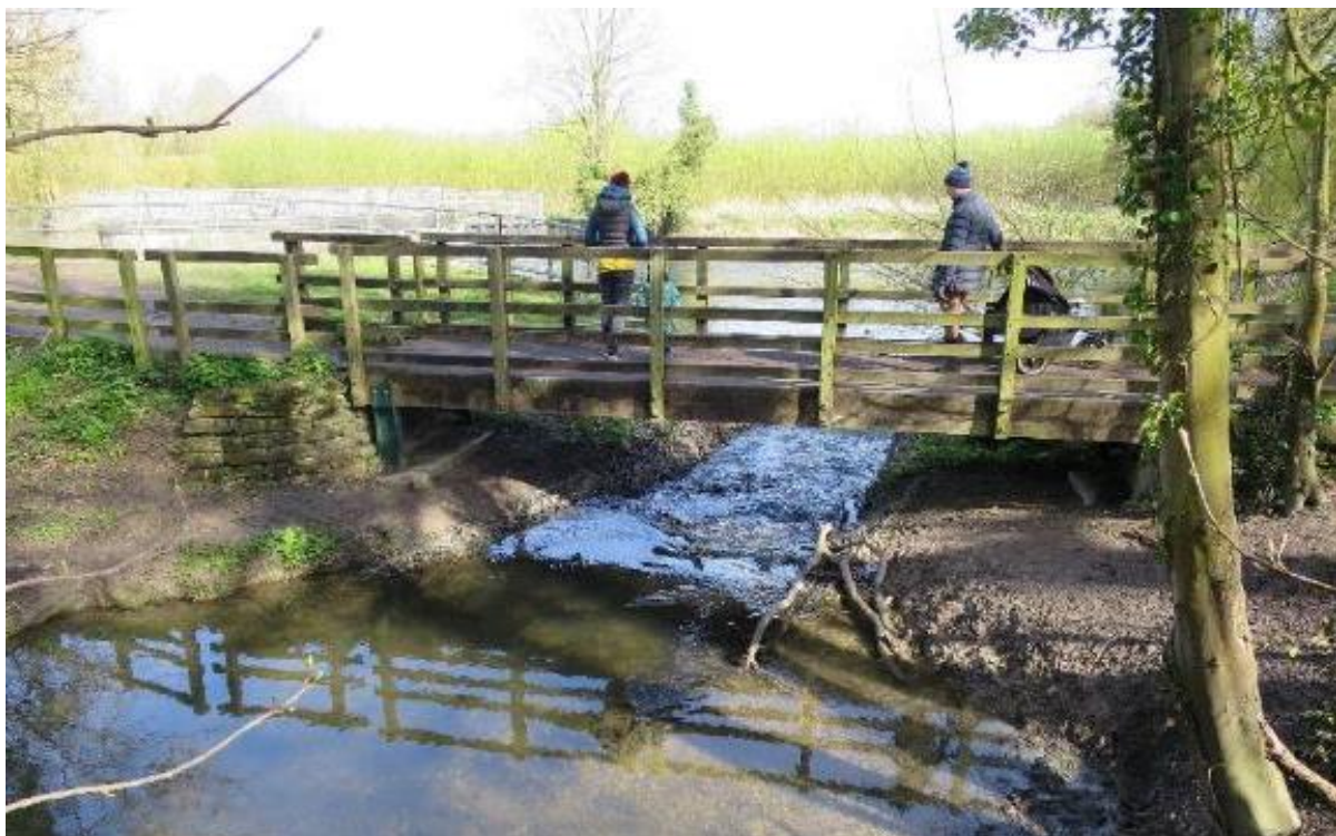
11. The Byron's Pool weir and sluice was constructed in 1949. This prevented fish from migrating upstream, however in 2011 a new cascading channel with pools and riffles was created to bypass the barrier providing an effective and attractive fish pass.
