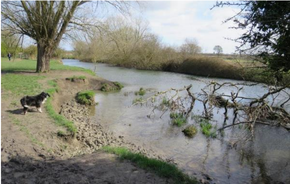
20. The riverbank has been damaged in a number of places by cattle, dogs and people. For several years some parts have been steadily eroded by cattle wading into the river to drink. Damage was exacerbated during the summer of 2018 because the three water troughs were out of use.
