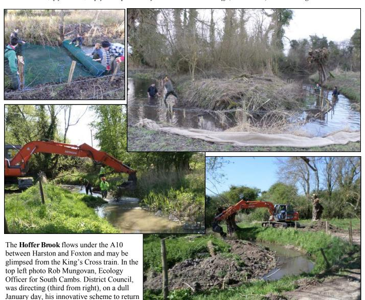
stream. The photo below the top left photo shows two grades of flint (gravel and small cobbles) being dropped into the channel (in April) creating a more 'natural' sinuous shape. This gravel is expected to increase species diversity by providing a home for invertebrates and a habitat for fish to spawn. The gravel/cobbles rest on plastic mesh to prevent their loss in the stretch where the silt is soft and deep. Immediately downstream, Ruth Hawksley, the Wildlife Trust's
